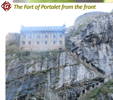
The Fort building is "pressed" against the cliff made up of thick, massive limestone beds (Devonian); the galleries allowing access from one level to another are built in fracture zones intersecting this series of beds. The architecture of this military building was designed based on the properties of the geological rock base.
